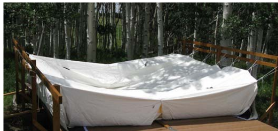
Tie the sidewall guy ropes to the lower side rail. (Step 2.)
