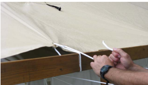
Tighten the guy ropes along the sides of the fly with the upper side rails. (Step 16.)
