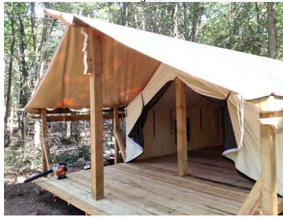
Custom tent frame by New England timber framer.
